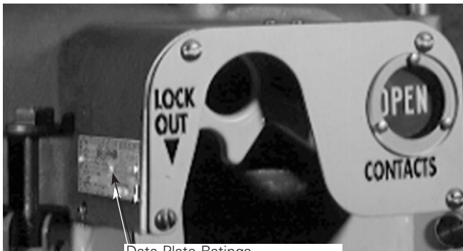
Figure 3. NOVA-TS triple-single recloser data plates are located on the sleet hood.
